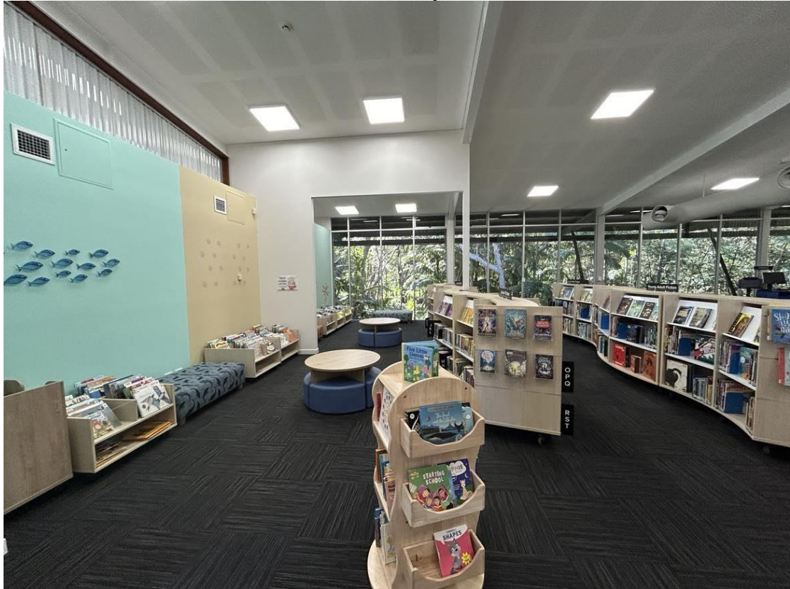
Image 5 Kingscliff Library after refurbishment: removal of enclosed walls to expand children's area.
